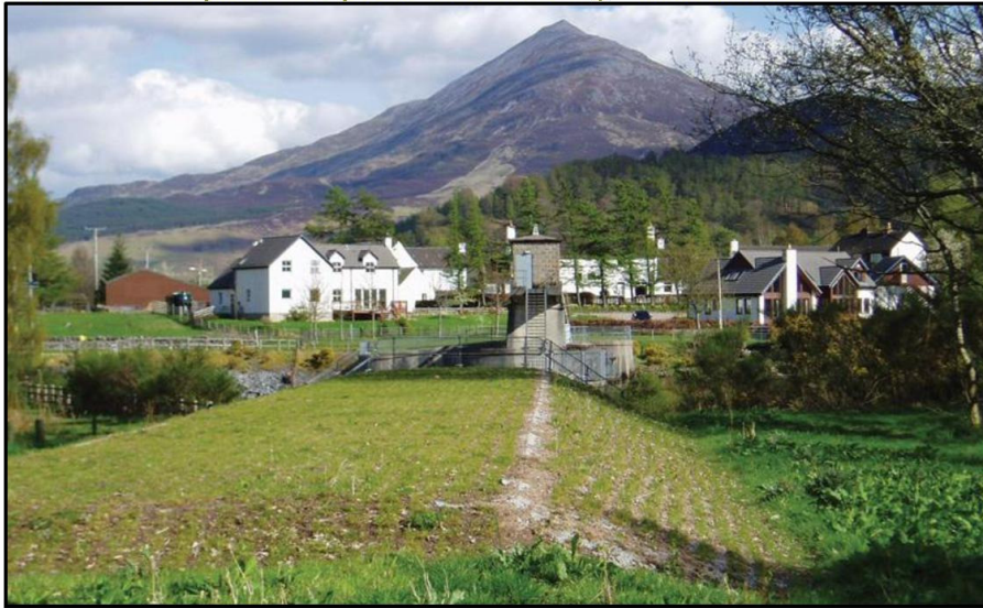
Photo 2 – Example of Completed Scheme using Voided Blocks
